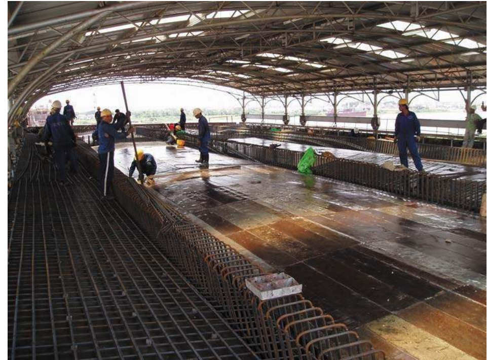
Preparation for concreting
