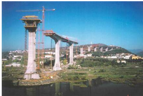
Regua Bridge, Portugal
