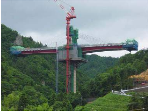
Rittoh Bridge, Japan
