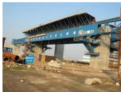
Transferring of Bracket
