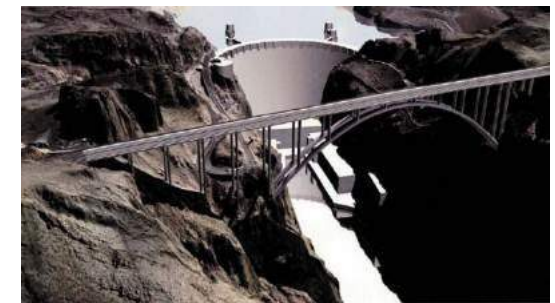
Colorado River Bridge, Se, USA ( Being constructed )
