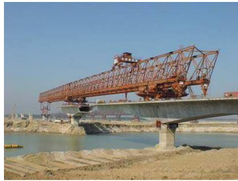
Paksey Bridge, Bangladesh
