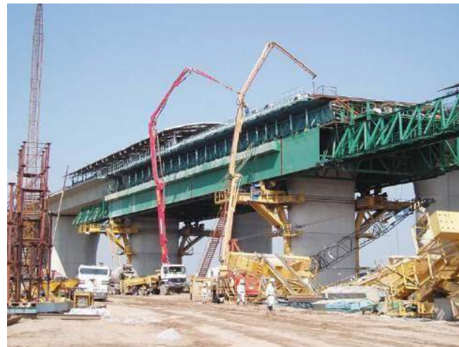
Red River (Thanh Tri) Bridge, Vietnam
