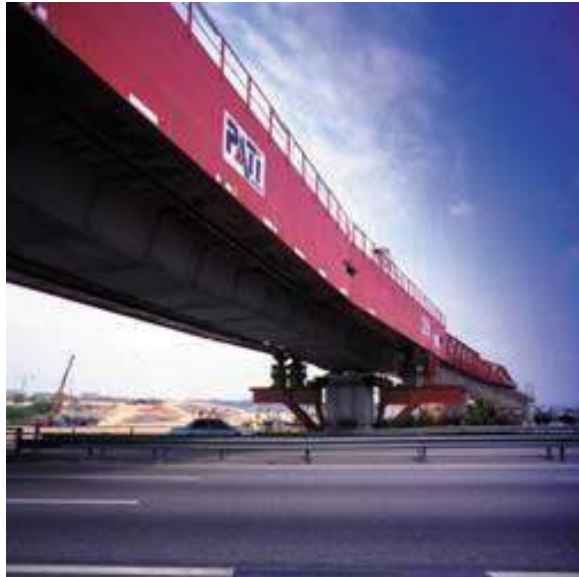
LRT2 Project, Malaysia (Hinged Gantries)
