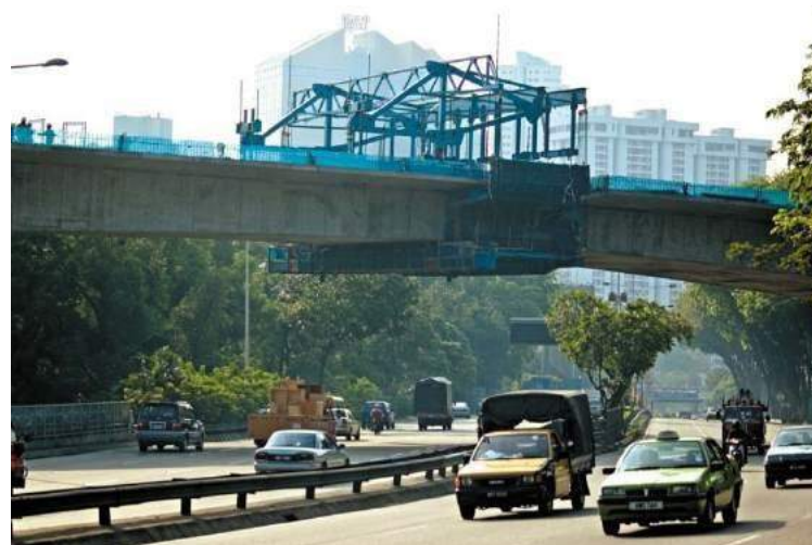
Bridge over Jalan Kuching, Malaysia
