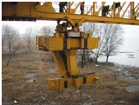
Transferring of Bracket
