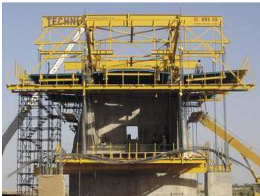
Khordad Bridge, Iran
