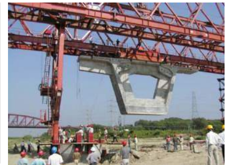
Paksey Bridge, Bangladesh
